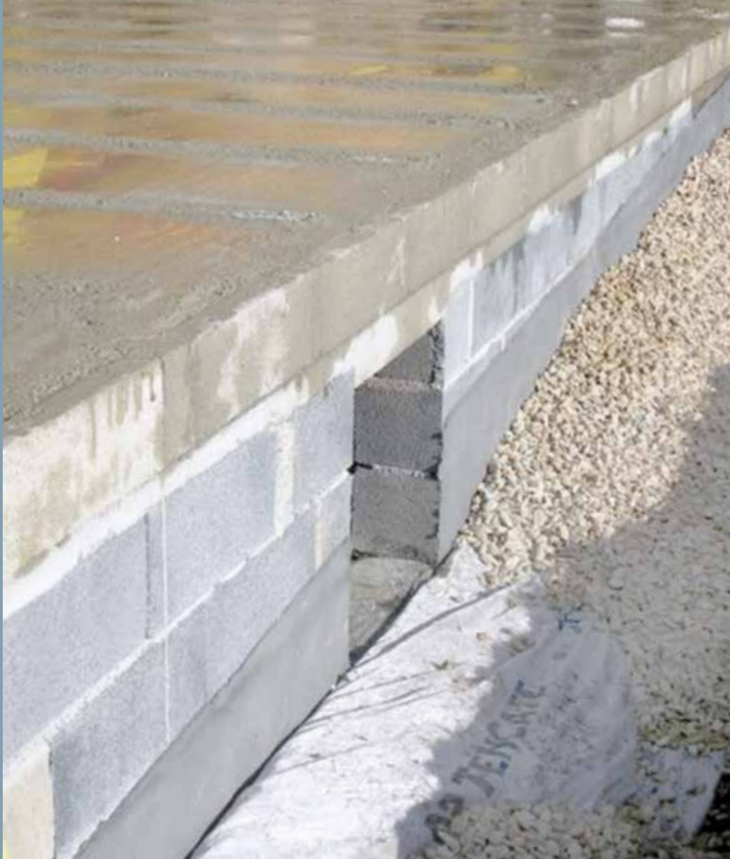
2022 LANKOFUGEANT applied to concrete blocks below ground.
